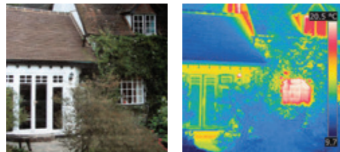
Above: The images show just how effective fitting energy efficient windows to your property can be. The right hand side of the property still has the original windows – the reds and pinks show heat escaping. However, the new extension on the left is fitted with energy efficient windows, the lack of reds and pinks proving they help dramatically reduce heat loss.
